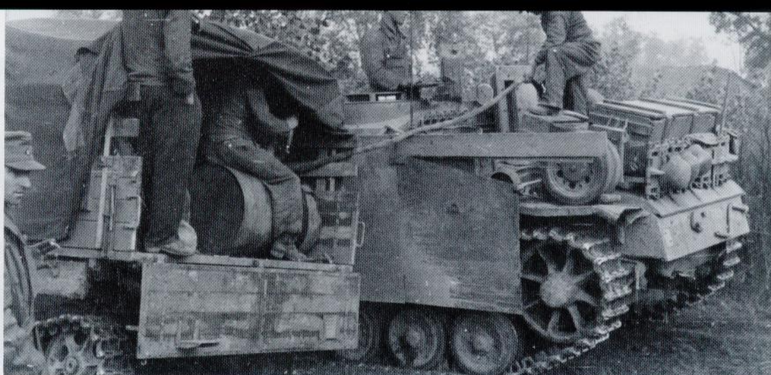
(Above) Refueling an armored vehicle in the field was often a tedious process. This StuG III of 286th StuG Brig is being refueled by a soldier operating a wobble pump mounted on a fuel drum. The StuG III is overall Dark Yellow, with a solid coat of mud on the side skirts. The unit emblem is Black crosses outlined in White on a Yellow background, with a Black outline.
