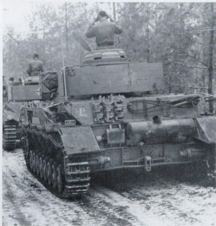
(Bottom right) A rear view of the same group of PzKpfw IVs shows the fading White division sign on the rear hull plate. Note the zimmerit paste applied to the rear turret skirting, and the overall Dark Yellow paint scheme. (Bundesarchiv)
