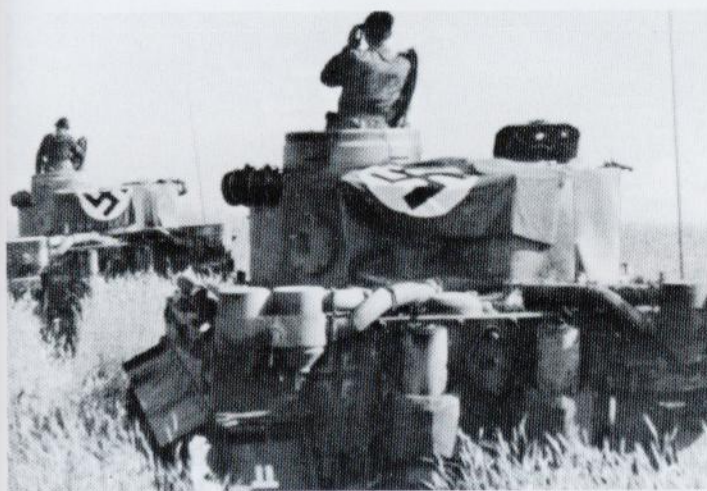
During the Kursk battle, German units fought in several towns and cities. This Tiger I of "Das Reich" is Dark Yellow with Red Brown and Olive Green mottling. The vehicle number is White. On the front turret side is the White gnome of the Tiger company. The Feifel air cleaners have been removed from this vehicle. (Bundesarchiv)
